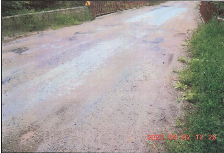
Photo 1: East Approach and Deck Top Looking West
