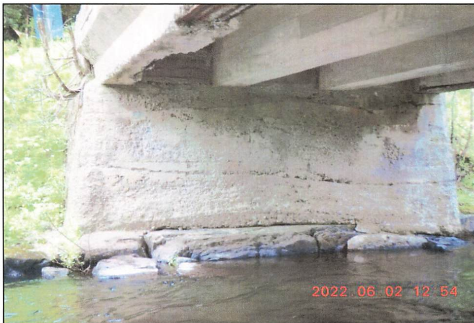
Photo 6: West Abutment Wall
