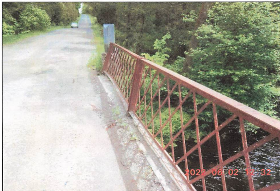
Photo 10: Outward Rotation of Southeast Barrier
