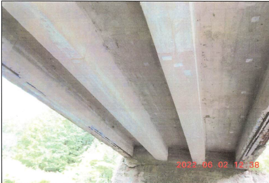
Photo 5: Interior Soffit and T-Beams Looking East
